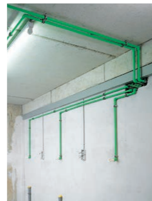
Surface installation
