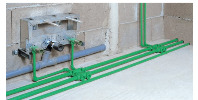
Floor distribution with distribution blocks
