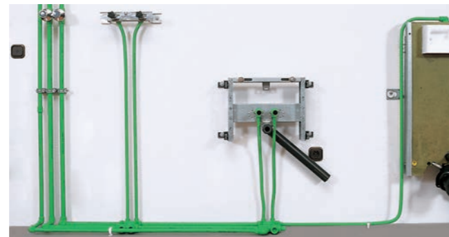
Surface installation
