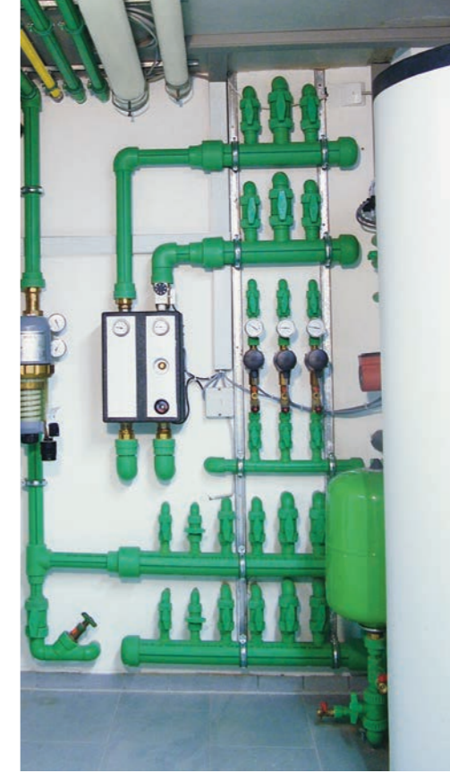
Distribution network for domestic water and heating in residential buildings
